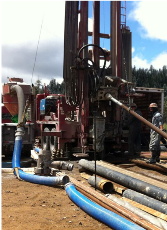
Figure 6: Geothermal Drilling Rig
